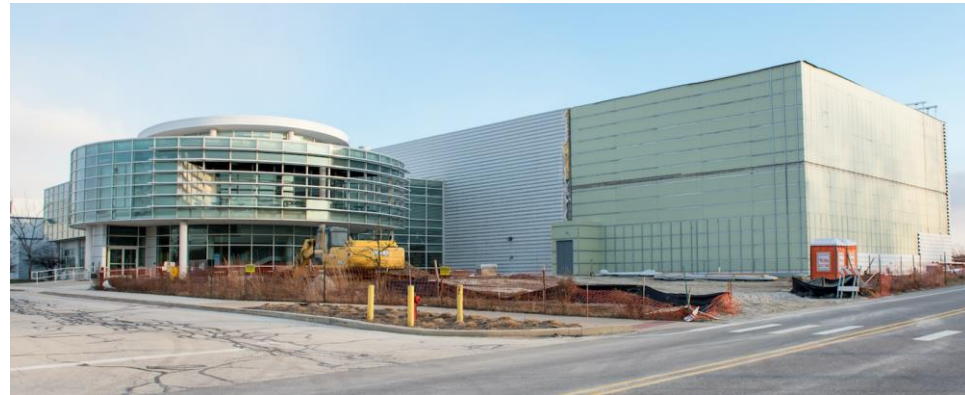
CNM Cleanroom Expansion
